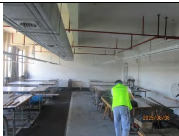
Work process 4 – edge painting
