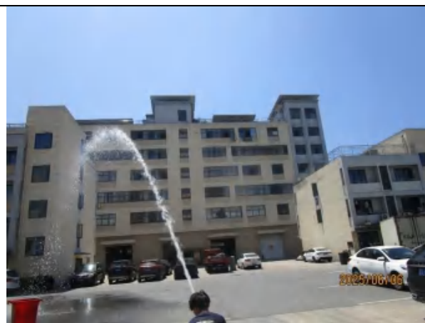
Fire hydrant testing
