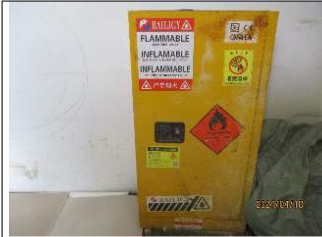
Chemicals stored in explosion-proof cabinet
