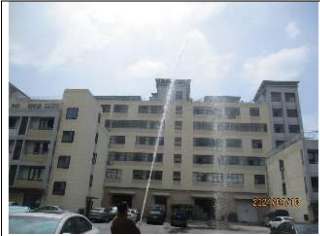
Fire hydrant testing
