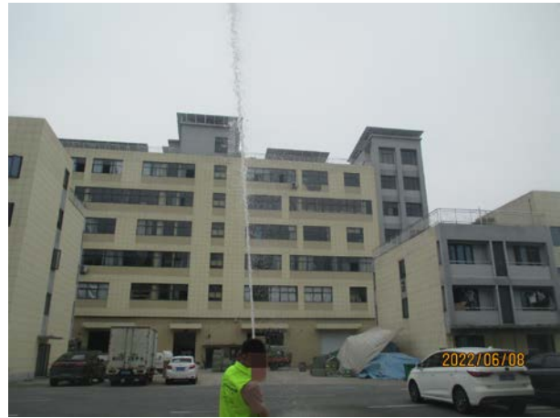
Testing fire hydrant
